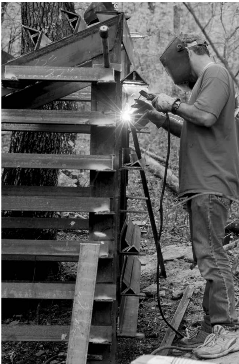
Figure 5.6 Building a bat gate above a sink opening. Photo by Danté Fenolio. (See Plate 21.)
